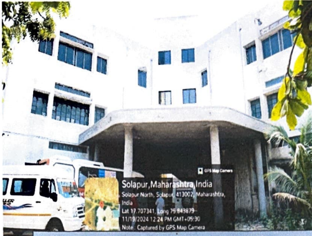
Front view of college building
